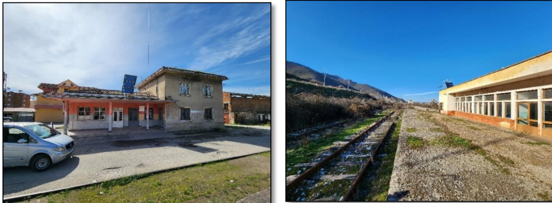
Figure 2-4 Railway stations of Peqin and Pogradec
