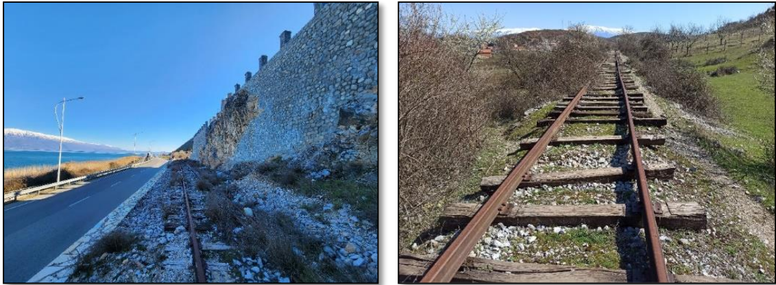
Figure 2-3 Railway line between Prrenjas and Pogradec
