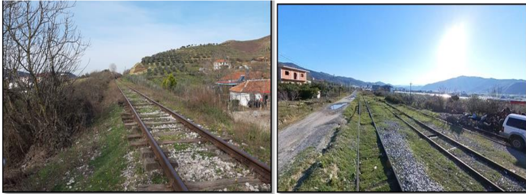
Figure 2-1 Infrastructure condition of the railway line between Rrogozhina and Elbasan
