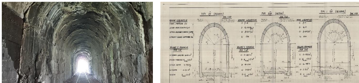
Figure 2-5: Existing railway tunnel of Qukës II and excerpt of old design
