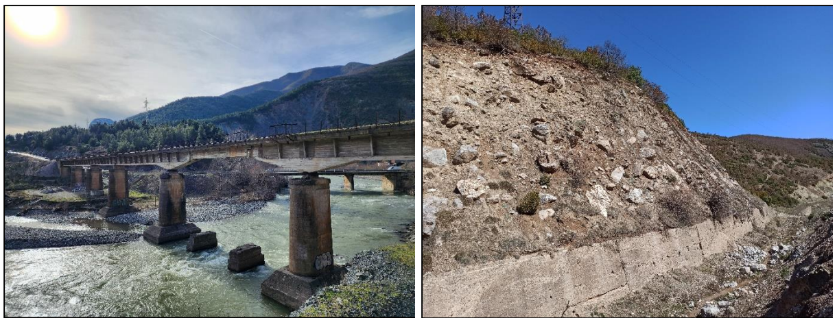
Figure 2-3: Railway line between Elbasan and Prrenjas
