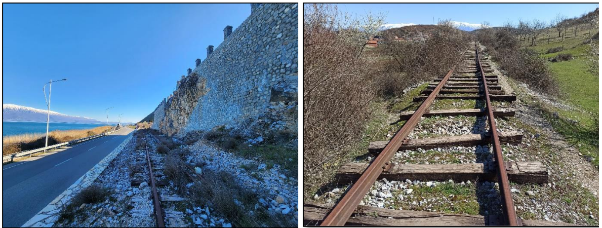
Figure 2-4: Railway line between Prrenjas and Pogradec
